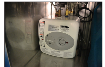
Water Heater Shown for 26CH Unit
